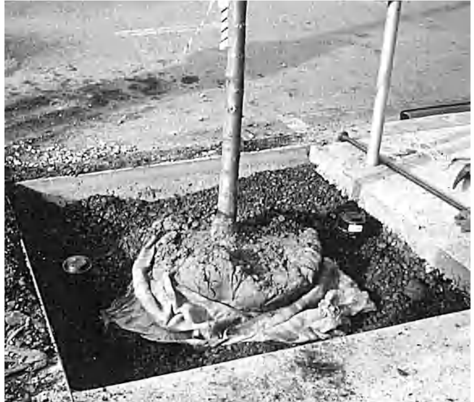
Fig. 18. Cutouts measuring 4 by 4 by 4 feet (64 cubic feet of fertile soil) are the minimum size for planting trees in sidewalks, patios, or parking lots. Pits measuring 5 by 10 by 4 feet are used in Philadelphia and other cities to plant large trees such as oak and sycamore.
