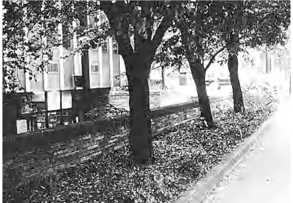
Fig. 22. Continuous planters provide good soil volume and can be covered with brick or cantilevered cement panels.
