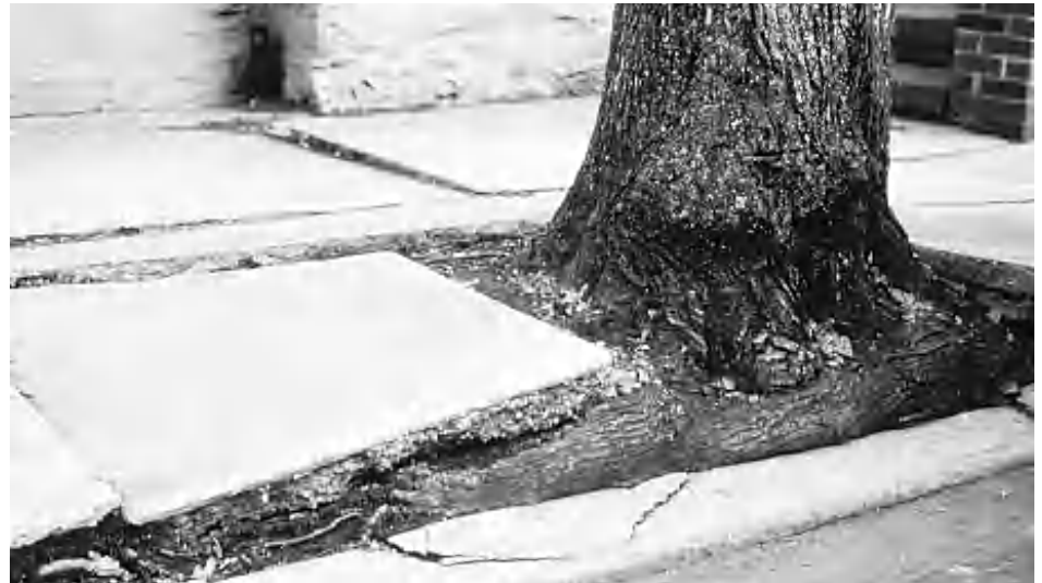
Fig. 2. Planting large trees in confined areas causes sidewalk and other damage.
