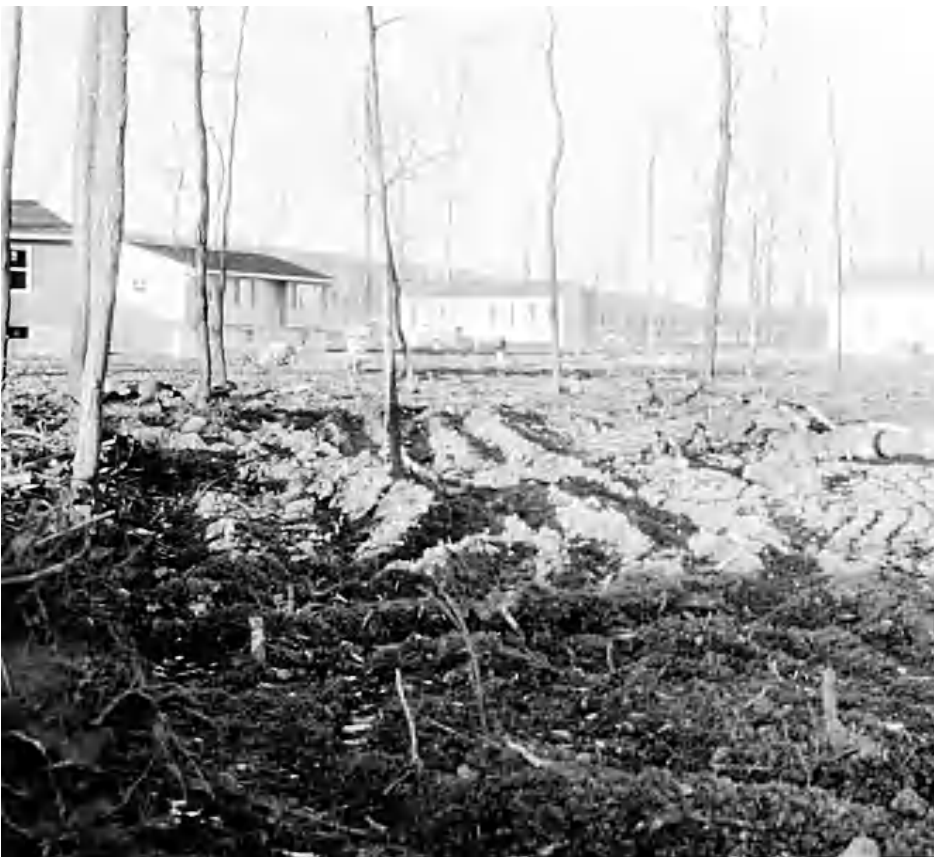
Fig. 28. Operating heavy equipment has ruined this soil. Soil structure must be protected to plant or preserve trees.
